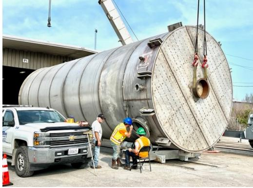
We continue to see more requirements for third-party passivation which is being performed above on a 40,000-gallon stainless steel API 650 shop-built tank.
